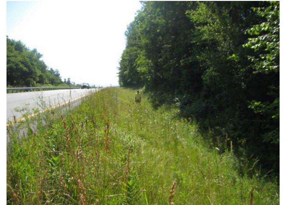
LOOKING UP SWALE FROM OUTLET
