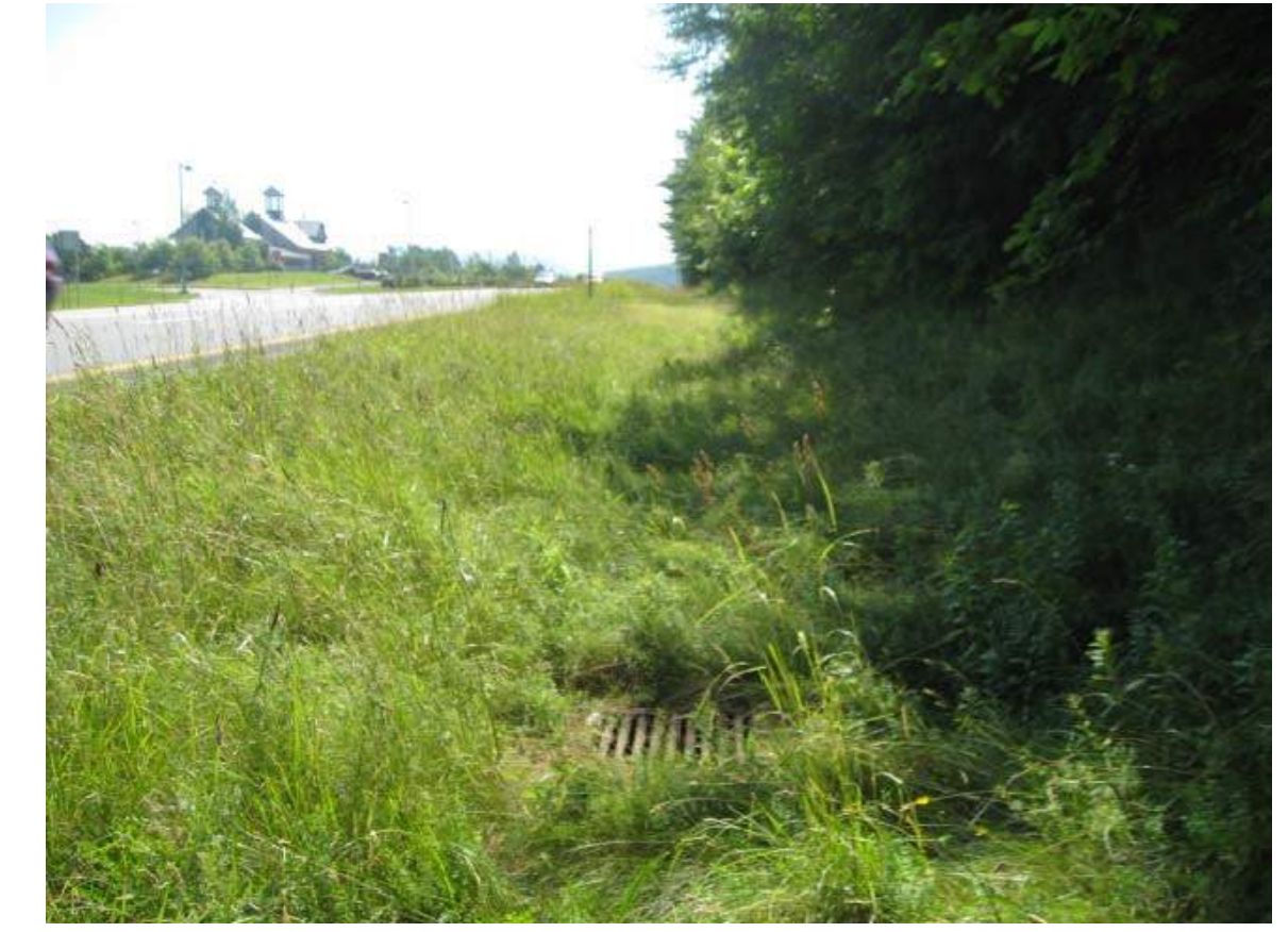
LOOKING UP SWALE FROM OUTLET
