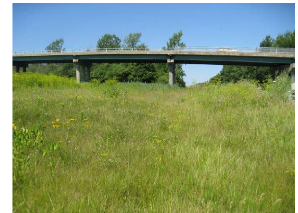
LOOKING UP WEST SWALE FROM CROSSOVER
